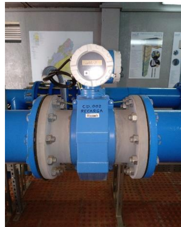
Figure 8. a) Recharge buster and bypass. b) Recharge electromagnetic flowmeter.
