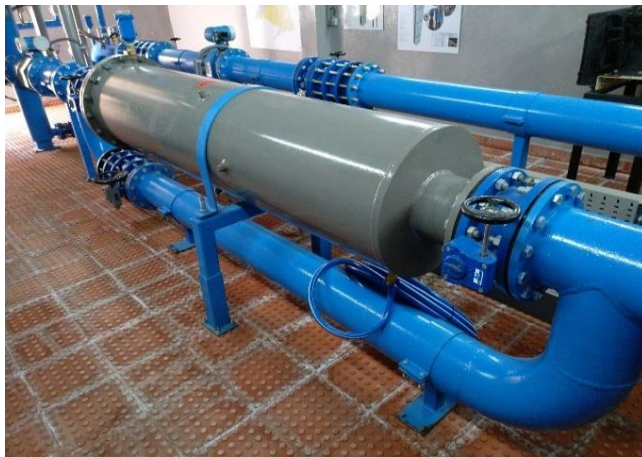
Figure 8. a) Recharge buster and bypass. b) Recharge electromagnetic flowmeter.
