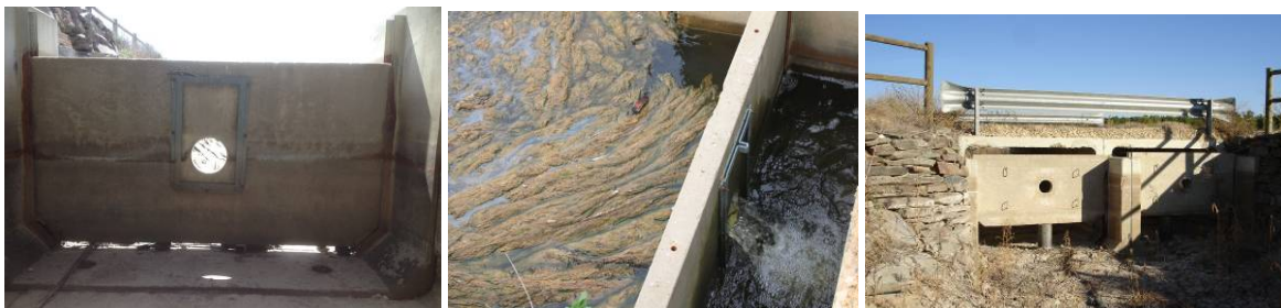
Figures 5-17 a) to c). Stopping and damming devices evolution in Arenales MAR experiences to mix water and to avoid its oxygenation.
