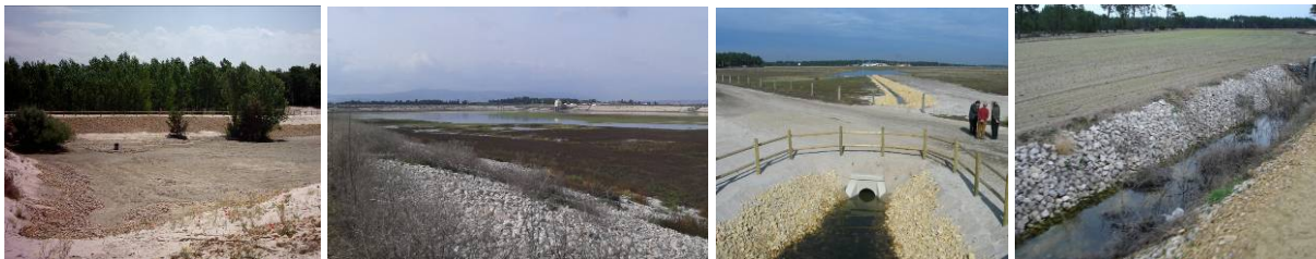
Figures 5-9 a) to d). Mudstone gravel filter to result in pH corrections as well as provide stability to some MAR facilities such as ponds (examples for Arenales and Menashe) and canals (Arenales).
