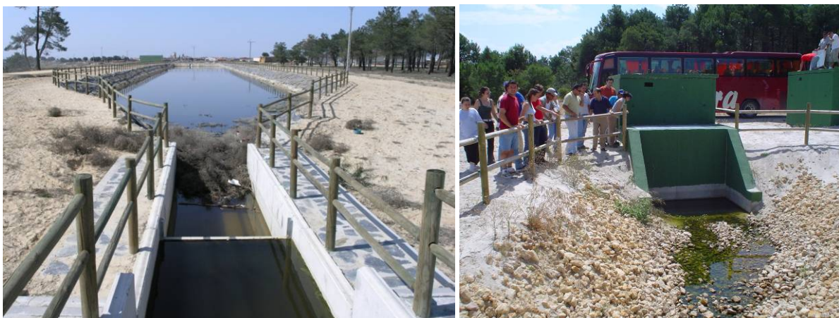
Figures 5-5 a) & b). Some examples for technical solutions already deployed in Carracillo council. Stagnation systems in the heading of some infiltration ponds; Arenales Aquifer, Spain.
