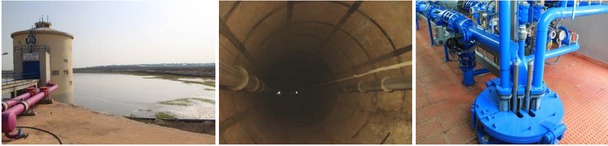
Figures 3-6 a to c). Specific designs for a huge infiltration pond in Shafdam, Israel (a); a MAR high diameter well (Maribor, Slovenia) and a dual system injection borehole (Madrid, Spain).
