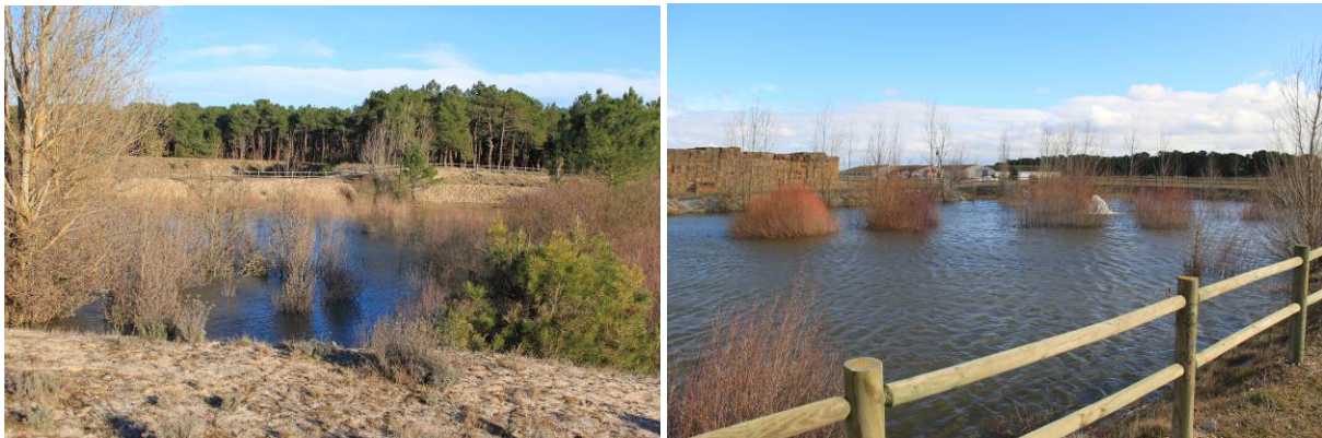
Figures 5-2 a) & b). Temporary storage of MAR water for decantation pre-treatment and recharge (heading infiltration pond) in Carracillo, Arenales Aquifer, Spain.
