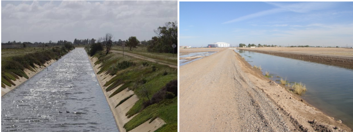
Figure 3-2 a) and b). Detailed studies of micro-topography in MAR channels in order to achieve a passive system in Adelaide (Australia) and Phoenix (USA).
