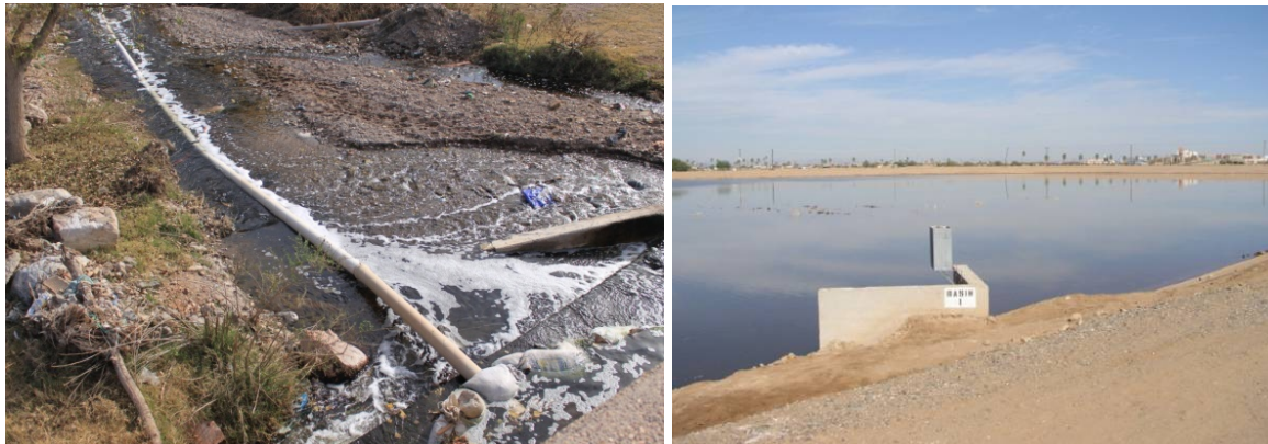
Figures 3-8 a) & b). Diversion from a river catchment directed at an infiltration pond (Chihuahua, Mexico) and control of the water thickness in an infiltration pond (Phoenix, USA).
