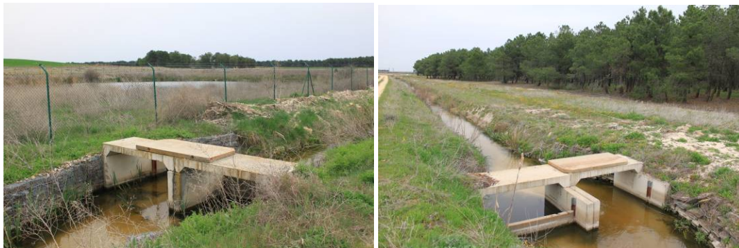
Figures 5-14 a) to d). Structure and system to facilitate the flow either below or in the middle of the weirs and precast concrete in order to mix the water stratification (a) and alternate opened gates in the double stopping devices to induce the mixing of water also laterally.
