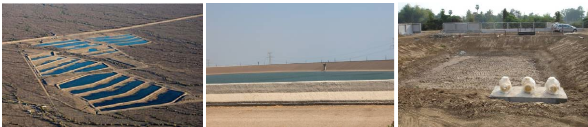
Figures 3-3 a) to c). Actions carried out on the morphology of infiltration ponds and channels. Studies of topography (a) and micro-topography to bring MAR water to infiltration wells by gravity, Castellón, Spain (b) and use of pumps to move water into an infiltration pond (active system) in the North of Thailand (c).
