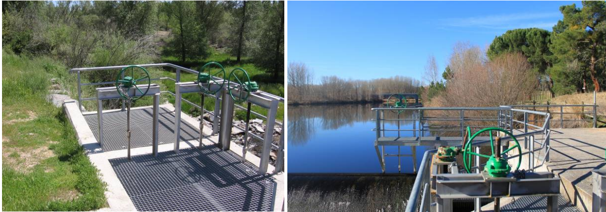
Figures 5-3 a) & b). Valves for manual control of the water volume diverted from the river to the canal for MAR activities in Santiuste basin, Arenales Aquifer, Spain.
