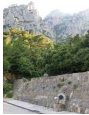
Figures 4-31: Perforated lamination and protection dam in a stream header to enhance the recharge in the aquifer and equipped with a tap for direct water collection. Tarragona, Spain.
