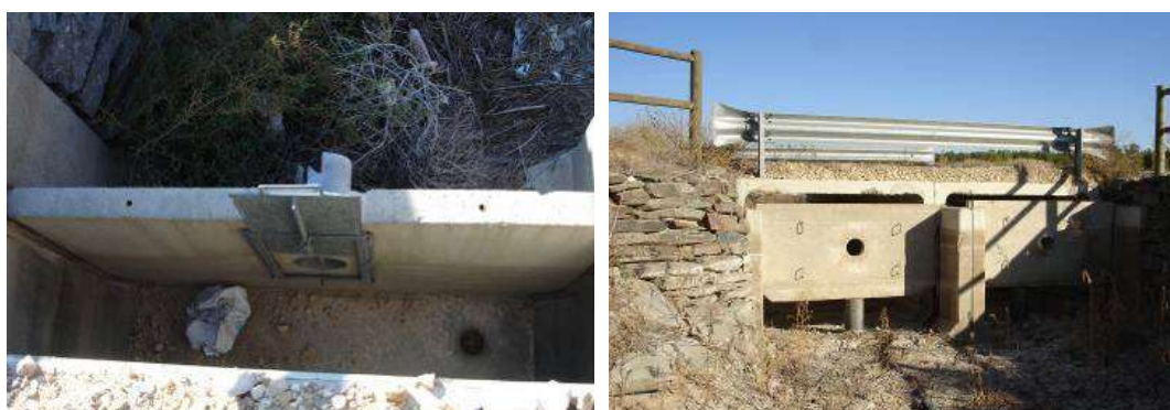
Figures 4-11 a & b: Elements (stopping devices) in the MAR canal. The locks (gates) are raised so the water flows either across the halfway drilled holes (a), underneath (b), or jumping over the slab so as to achieve a running water homogenization.
