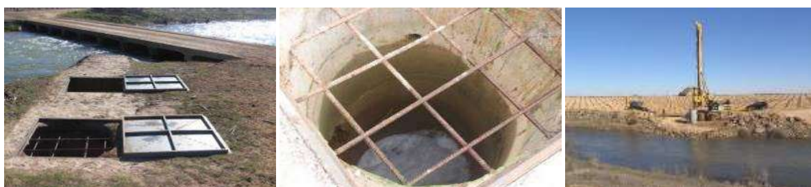
Figures 4-44 a to c: Deep well for MAR next to Guadiana River's canal (Spain).
