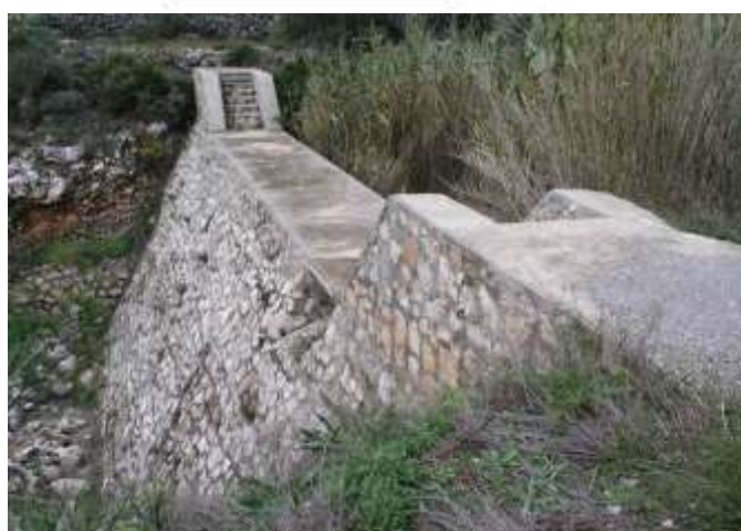
Figures 4-26 a & b: Dam diagram (a) and example for a dam specific for MAR and lamination in Alicante province, Spain.
