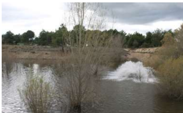
Figure 4-6: West Infiltration pond in Carracillo District, Los Arenales demo-site (Spain).
