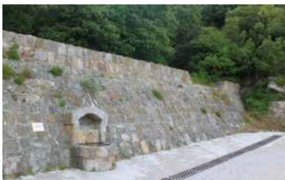
Figures 4-31: Perforated lamination and protection dam in a stream header to enhance the recharge in the aquifer and equipped with a tap for direct water collection. Tarragona, Spain.
