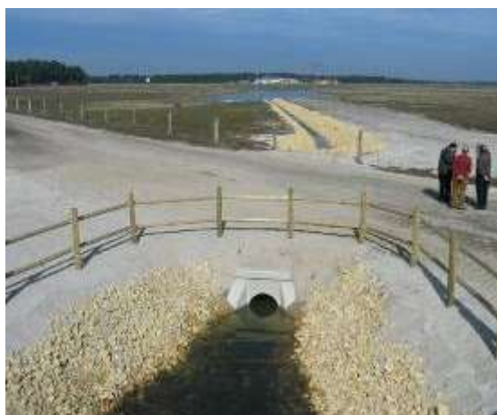
Figure 4-5: Infiltration pond in Carracillo District, Los Arenales demo-site (Spain).
