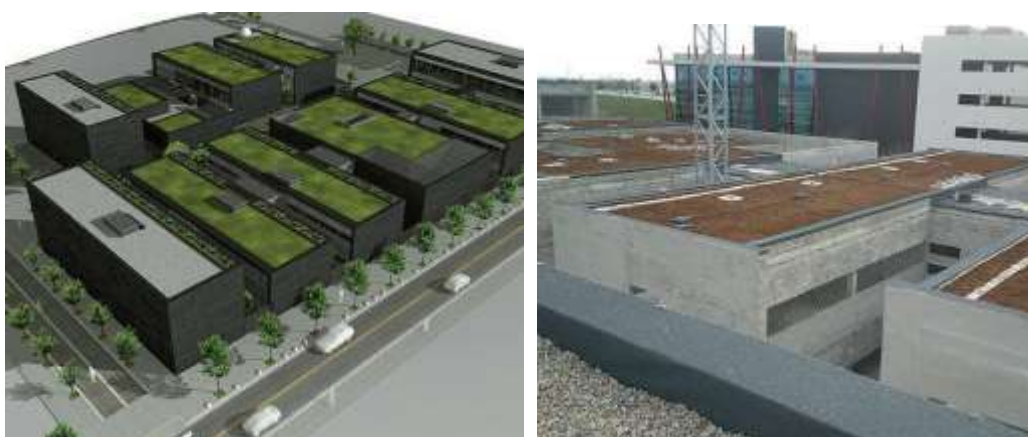
Figures 4-65: Model and construction process of the green roof of the Parc Bit building, Palma de Mallorca (Spain).
