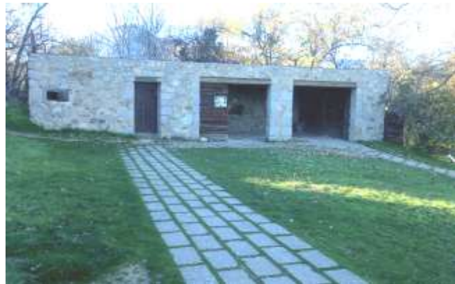
Figure 4-72: Discontinuous permeable paving.
