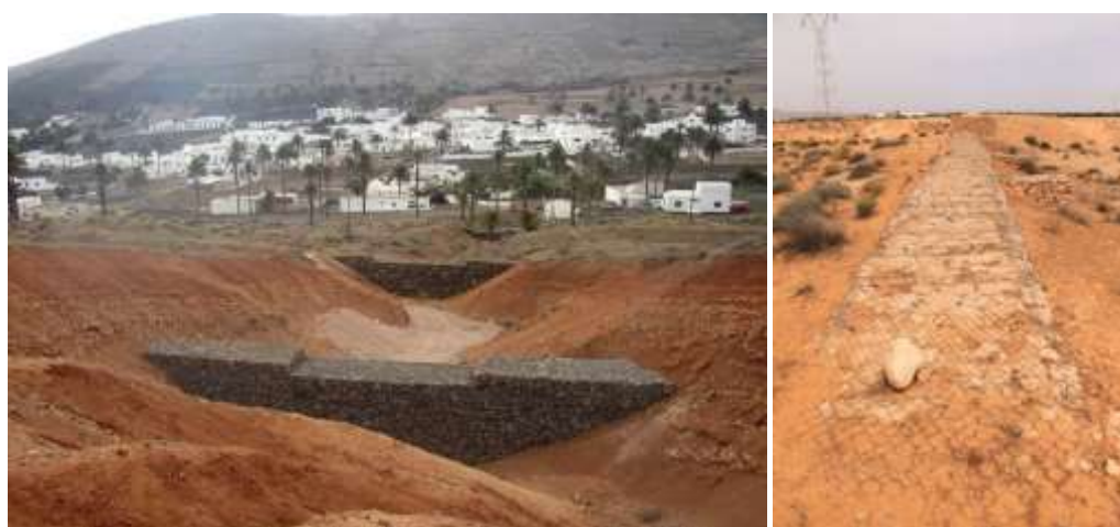
Figures 4-29: Gavions block reservoir dam in Las Palmas, Canary Islands (Spain) and check dam near Zarzis (Tunisia).
