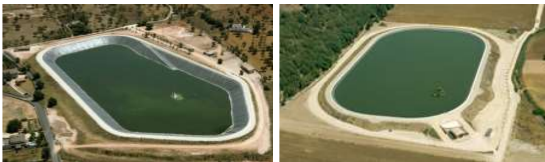
Figures 4-20: Irrigation ponds of reclaimed water in Majorca island, Spain.
