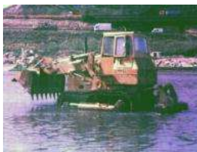
Figure 4-32: Riverbed scarification in Barcelona (Spain).
