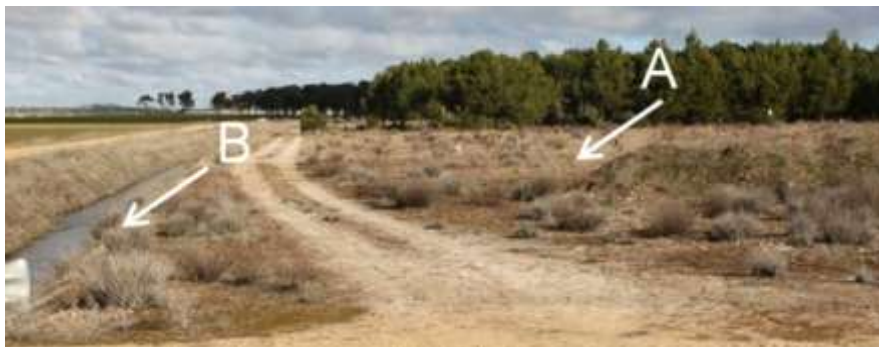
Figure 4-40: Old well filled with sand and gravel (A) and in pipe connection next to a MAR canal (B). Invisible recharge at Los Arenales demo-site, Spain.
