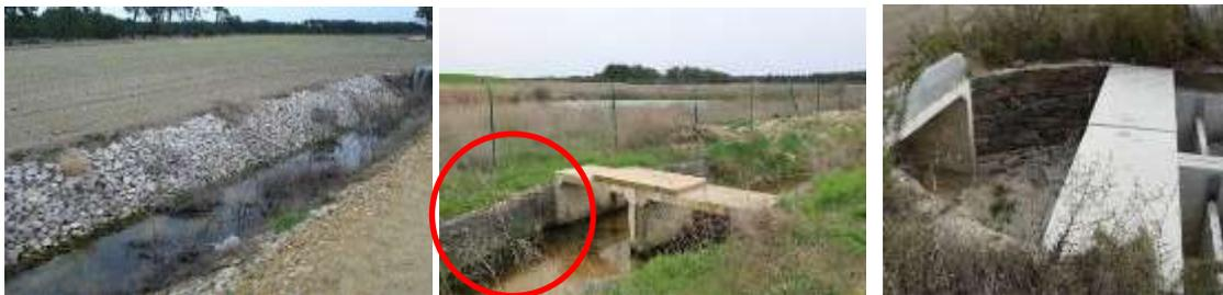
Figures 3-17 a to c. Mudstone gravel filter to induct pH corrections in MAR water as well as provide stability to some MAR facilities such as ponds (Santiuste, Los Arenales aquifer) (a & b). Protection gabions in the bottle neck between the MAR canal and a stopping device (c).
