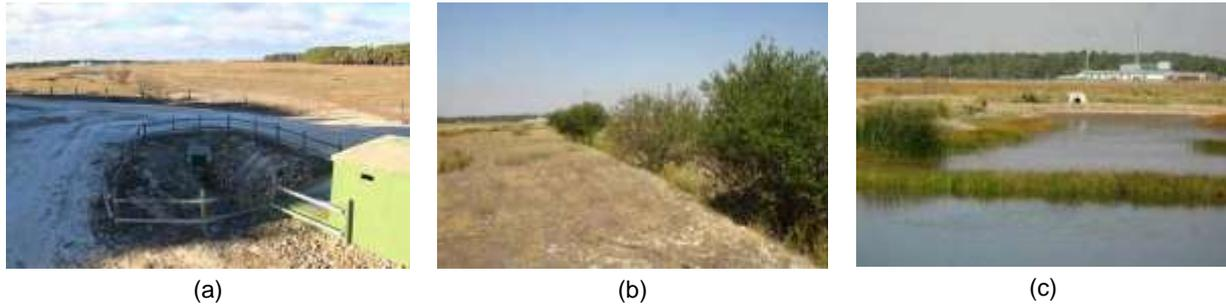
Figure 3-37: El Carracillo "Triplet" composed by an infiltration pond surrounded by a piezometer network (left), a bio-filter in the MAR channel (centre) and an artificial wetland (right) prior a spreading area for infiltration.
