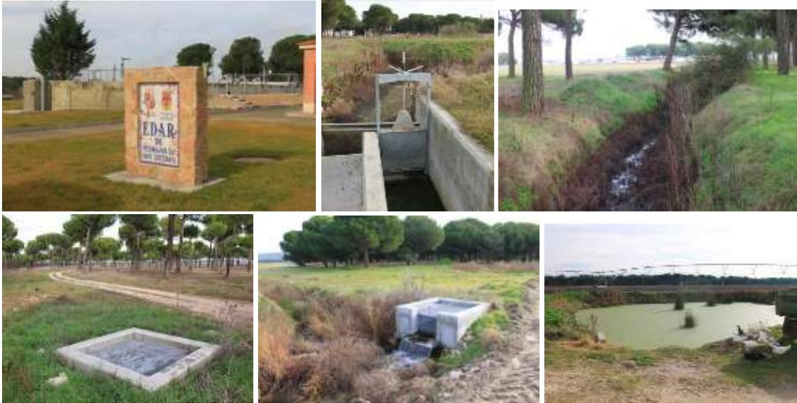
Figures 3-45 a to f: Alcazarén MAR system´s singular points: Pedrajas WWTP (a); connection point where converge water proceeding from the WWTP, runoff and Pirón river diversion pipe (b); runoff canal proceeding from Pedrajas village (c); spillway (d); valve 2 monitoring cage (e) and final sandpit used as a infiltration pond (A.W. 2) (f).
