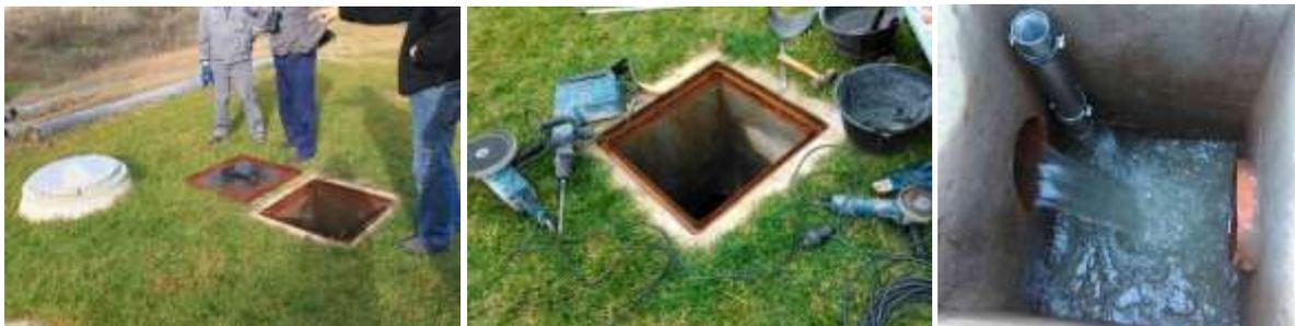
Figure 3-47: WWTP casket at the exit of Pedrajas de San Esteban WWTP (a), modifications for the gravel box (b) and preparation of the filter box and double spillway after the WWTP (c). 2016, February.
