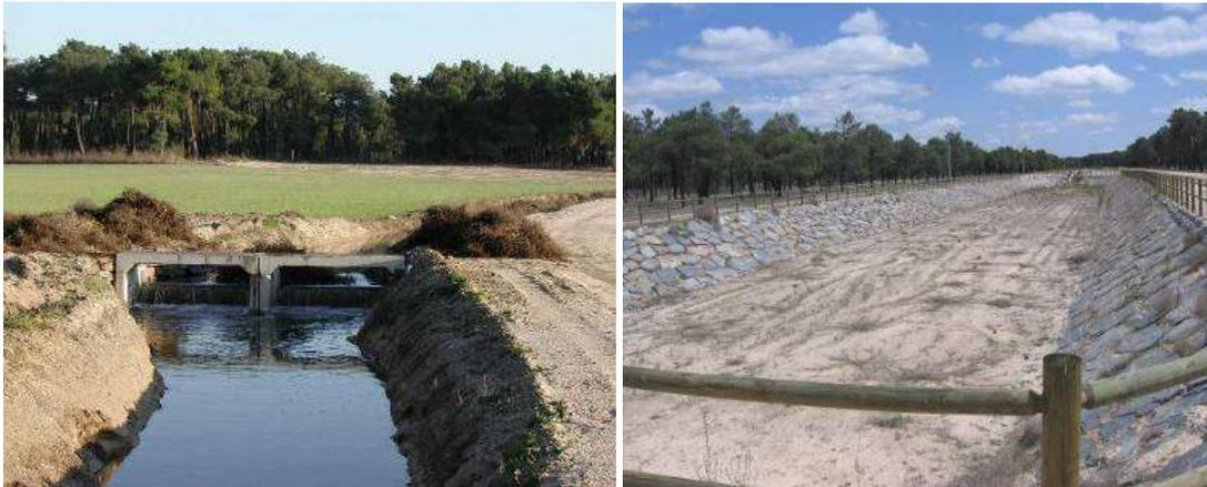
Figures 3-15 a & b: 2H/3V design (a); 3H/2V as the most common slope in the channels and ponds borders for Los Arenales environmental conditions (b).
