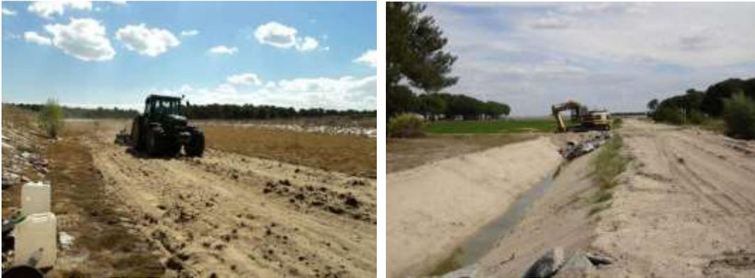
Figures 3-20 a & b: Cleaning and maintenance operations in ponds and canals by means of excavators (clogged sand is replaced by clean sand (a), and scarification by means of excavators with specifically adapted accessories (b)).
