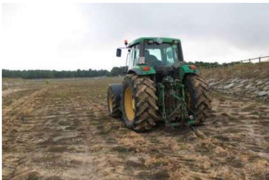
Figure 3-10: Tractor ploughing the surface of Santiuste Basin’s head infiltration pond.
