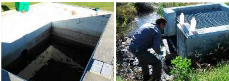
Figures 3-54: Alcazarén area. DBP test dropping hypochlorite at the exit of the WWTP, samples collection at valve 1 point and determination *in situ* of unstable parameters.
