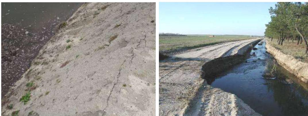
Figures 3-14: a & b. 1H/1V slope in MAR canals with potential slices due to desiccation processes (a); example for landslides impact in Santiuste MAR canal curves (b).
