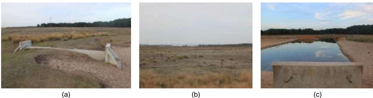
Figure 3-38: El Carracillo "Triplet" last elements: spillway (a) to pour water from the artificial wetland into the spreading infiltration field (b). Triplet seen from the spillway to the heading direction (c).
