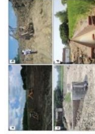
Figure 3(a) Excavation of pond, (b) drilling of recharge wells, (c) modified recharge well for measuring flow rates (non-modified wells are seen behind), and (d) drain constructed to divert wastewater from households away from the pond.
