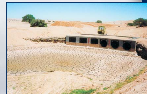
Looking in a downstream direction, pre-sedimentation basin in front of the flow divider with infiltration basin B in the background. (S. Zeelie, 1997)
