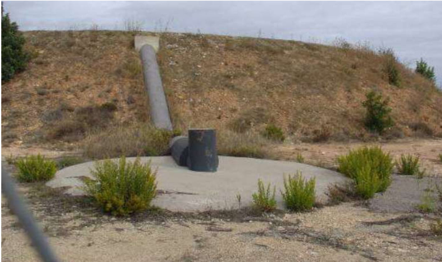
MAR borehole associated to an Irrigation pond
