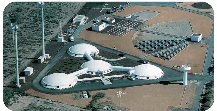
Reverse osmosis waste water treatment plant.
