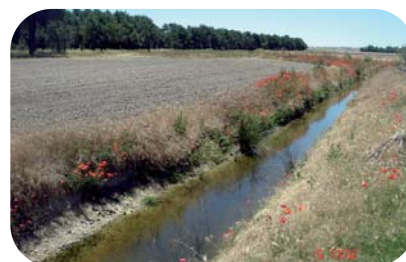
Picture of the infiltration pond and artificial recharge channel of the Cubeta de Santiuste facility (Segovia).
