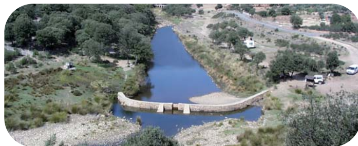
Small dam to reserve water in Cabañeros. (Photo: TRAGSATEC).
