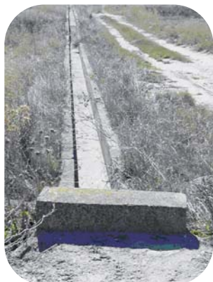
Drainage ditch on a hillside. The collection of rainwater reduces erosion and enables greater use of the runoff water. Navarre. (Photo: TRAGSATEC).
